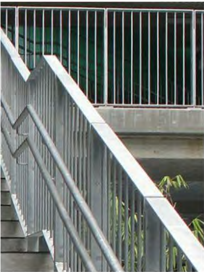
7 METAL BALUSTRADE / NEW FENCE FINISH: HOT DIP GALVANISED
