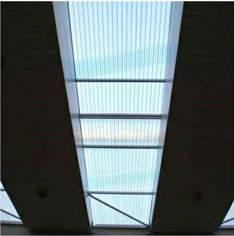
4 POLYCARBONATE ROOF SHEETING - SIMILAR TO EVERBRITE
