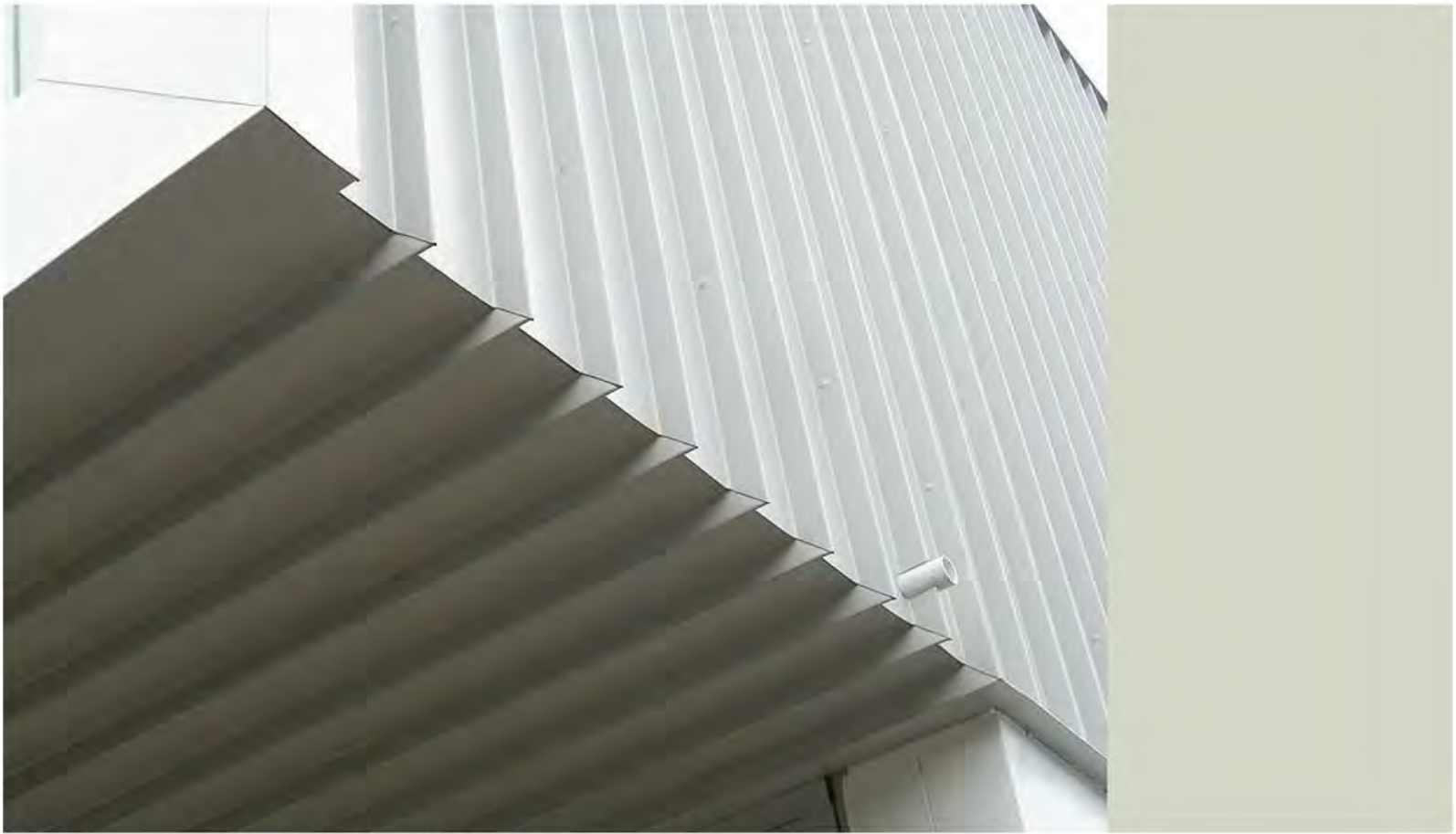
3 MAIN ROOF SHEETING - LYSAGHT LONGLINE 305 COLOUR: COLORBOND SURFMIST
